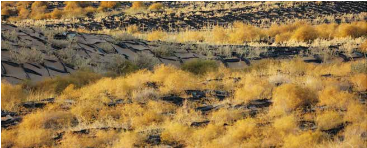
京新高速公路沿线防沙固沙成效显著 Significant success achieved in sand prevention and fixation along the Beijing-Xinjiang Expressway
