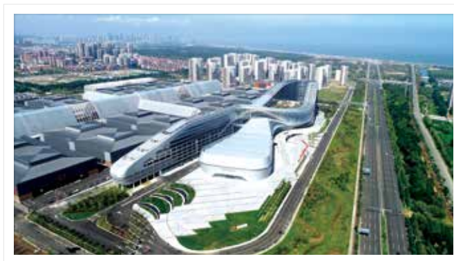
中铁青岛世界博览城会议中心综合体项目侧视图 A side view of the China Railway Qingdao World Expo City Convention Center complex project
