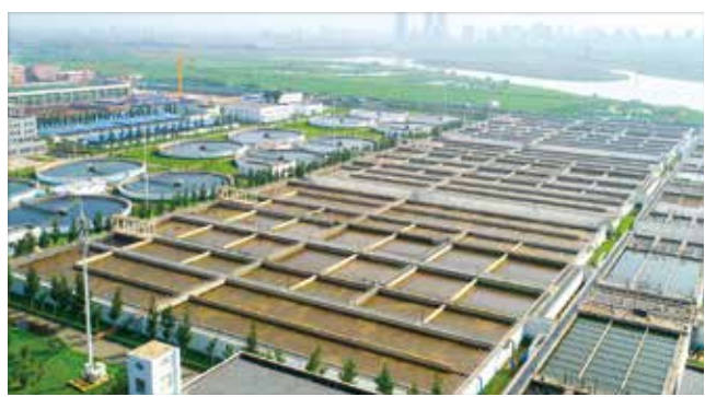
长春市北郊污水处理厂扩建及提标改造工程新建厂区西侧鸟瞰 A bird's eye view of the west side of the new plant area of the Beijiao Sewage Treatment Plant extension and upgrading project in Changchun
