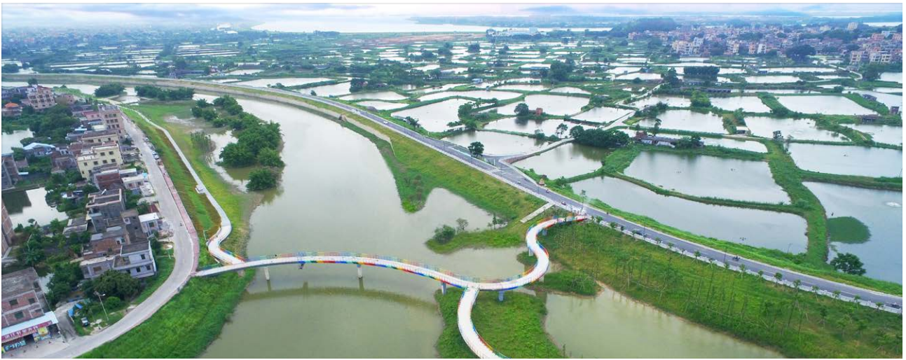
● 中铁上海局承建的鹤山市沙坪河综合整治工程 Comprehensive regulation project of shaping River in Heshan City undertaken by China Railway Shanghai Group Co., Ltd
